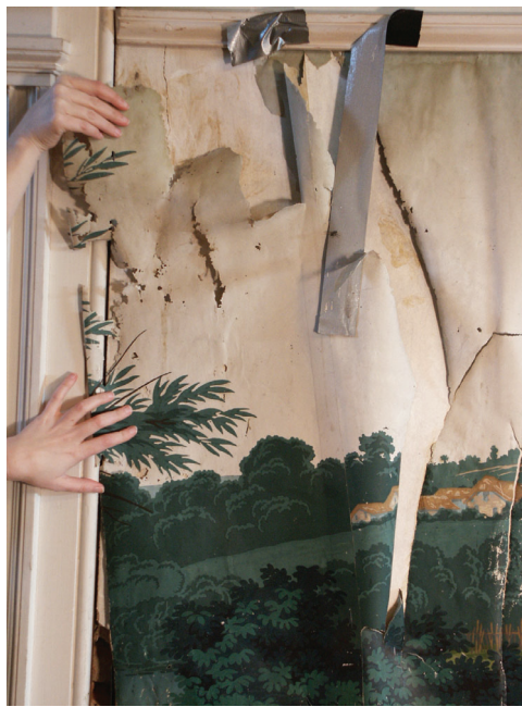
Fig. 4. Tears, insect predation, embedded grime, discoloration from contact with rubber cement, and duct tape
