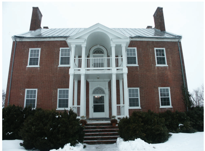
Fig. 1. Willow Wall, Old Fields, West Virginia
