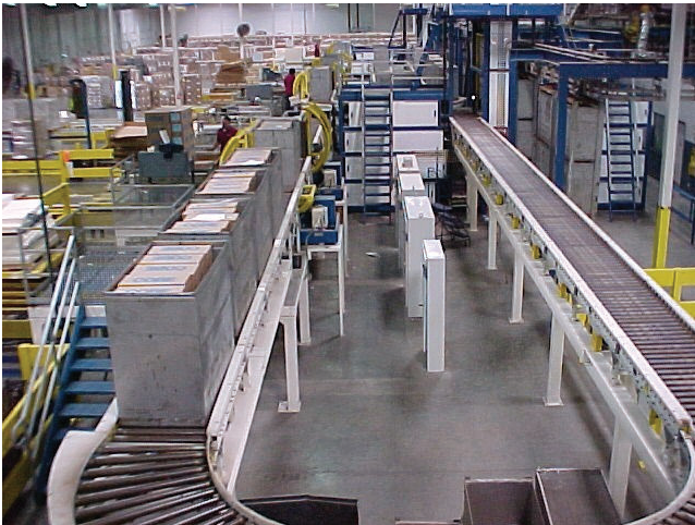
Fig. 12. Conveyor leading to gamma radiation facility, Corona, California
