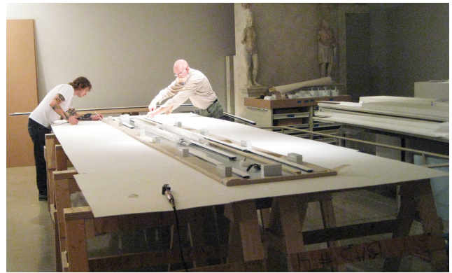
Fig. 5. Mounting one of the sixteen foot watercolors to an aluminum honeycomb panel in the Kelsey Museum galleries
