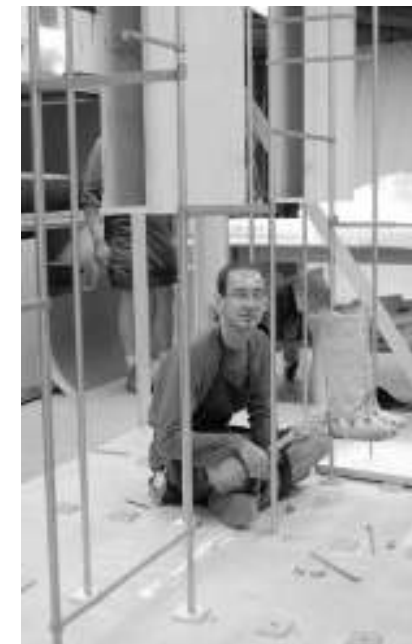
Mount construction in progress.
